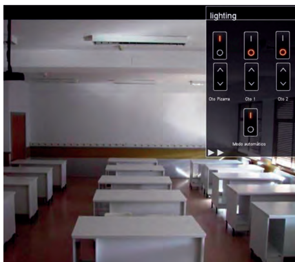
The project tested a range of techniques, including integrated control of lighting (pictured)
